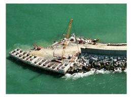
**(b)** Installation of the OWC power plant on the breakwater.
