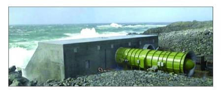
**Figure 2.14:** LIMPET OWC device from the Isle of Islay, Scotland, United Kingdom (Heath, Whittaker, and Boake, 2000).
